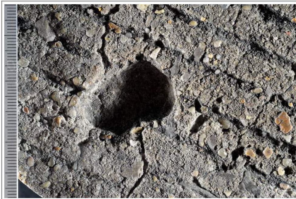
Figure C4. Photograph of top of core showing pit; scale in millimeters.
