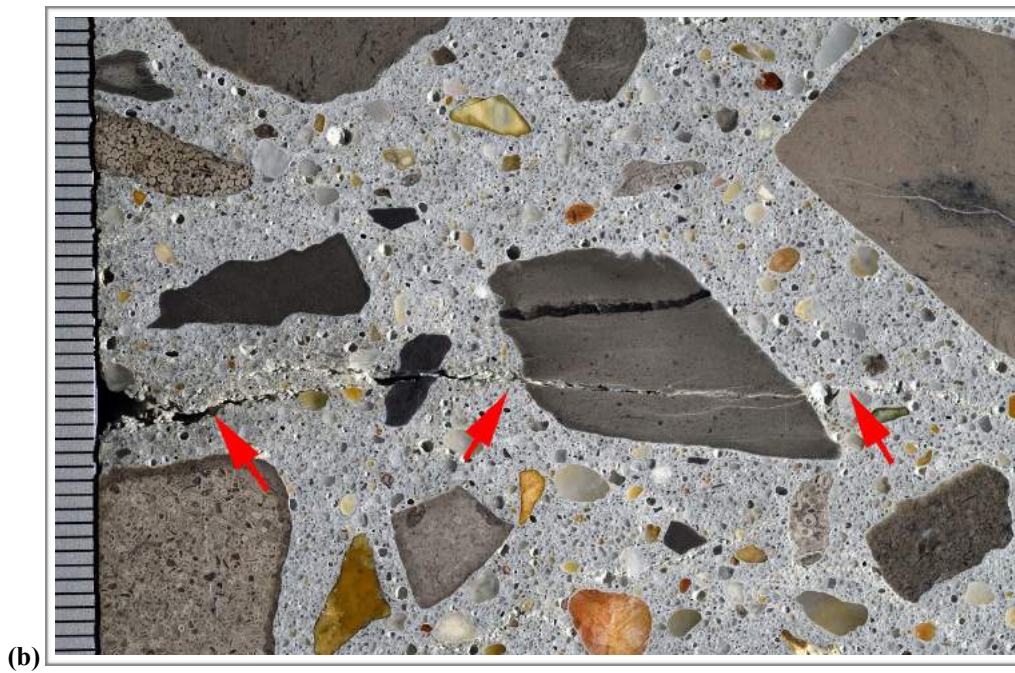
Figure A7. Photographs of the polished surface showing sub-horizontal cracks (red arrows) at (a) 75 mm (3 in.) and (b) 110 mm (4 3/8 in.) below the top surface.
